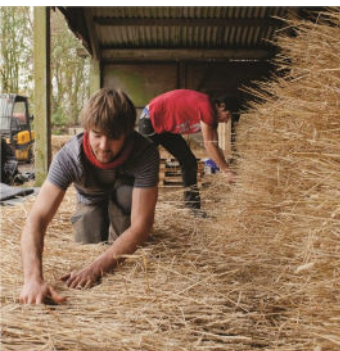
Thatchers at work constructing the cladding panels in their workshop
